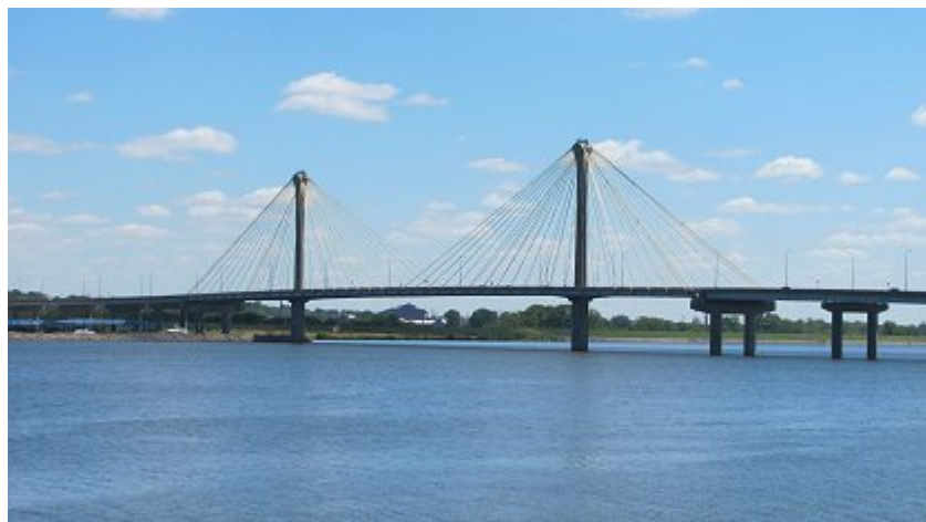
Photo of the Clark Bridge
